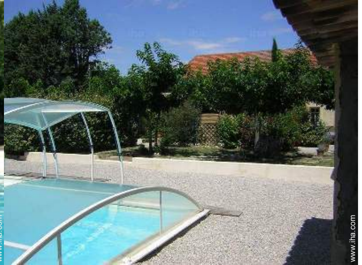
Covered swimming pool
