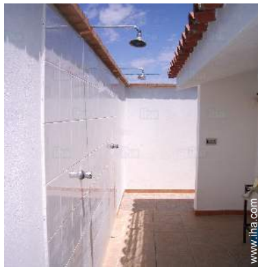
outside shower facilities
