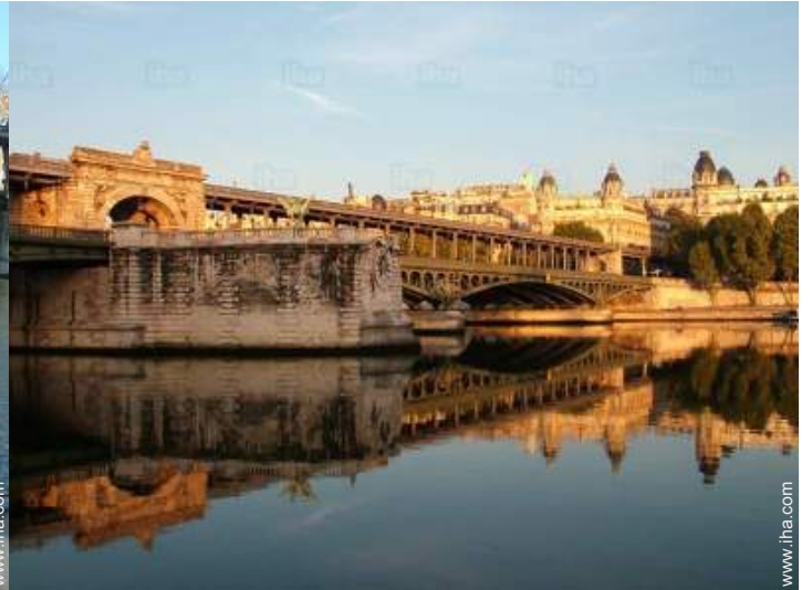
view over the river
